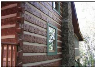
Custom 6x12 Log Home with Edge Chamfer for a rustic Antique look.
